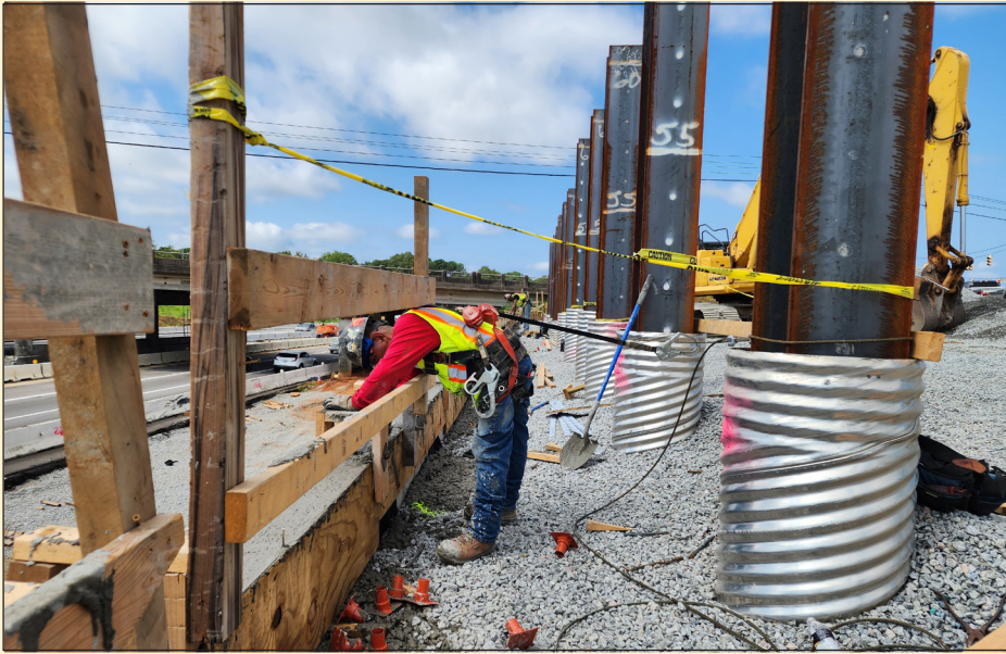
Carlos Zuniga, concrete finisher for CRG, Inc.
