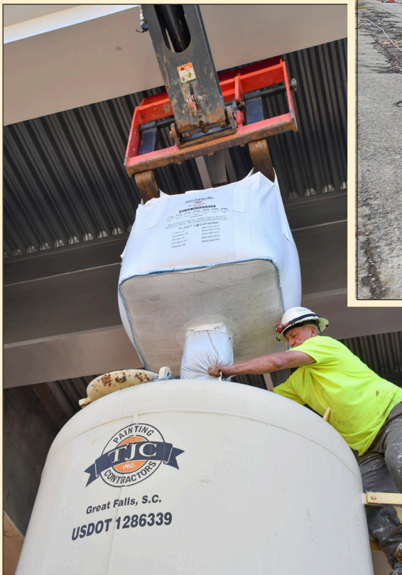
Mike Burchell, TJC Painting Contractors, Inc. painting new bridge structure SC-267.
